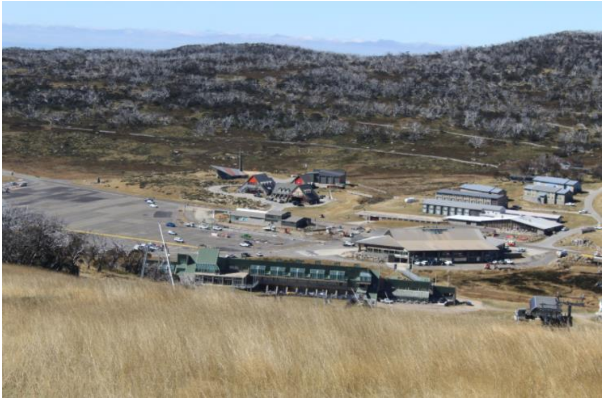
Figure 10: View looking towards an existing telecommunications facility from adjacent to the Village 8 Express Chair Lift Station
