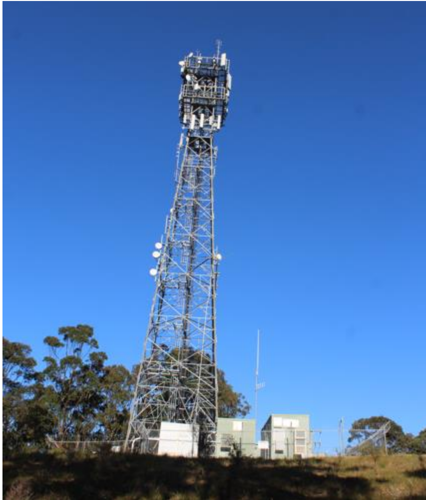
Figure 7: By contrast to the Proposal, an existing telecommunications facility using a lattice tower instead of a monopole
