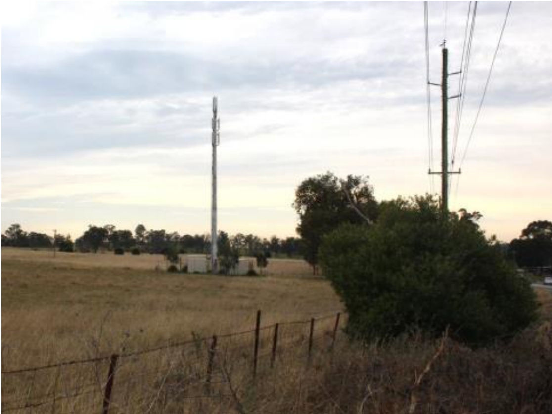
Figure 9: Similar to the Proposal, an existing telecommunications facility using a monopole and turret or collar mount antenna arrangement.
