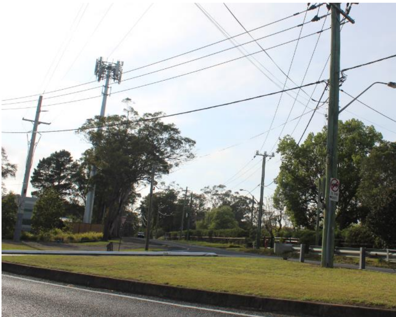
Figure 8: By contrast to the Proposal, an existing telecommunications facility using a monopole with a square headframe located at 43 Cattai Ridge Road, Glenorie.
